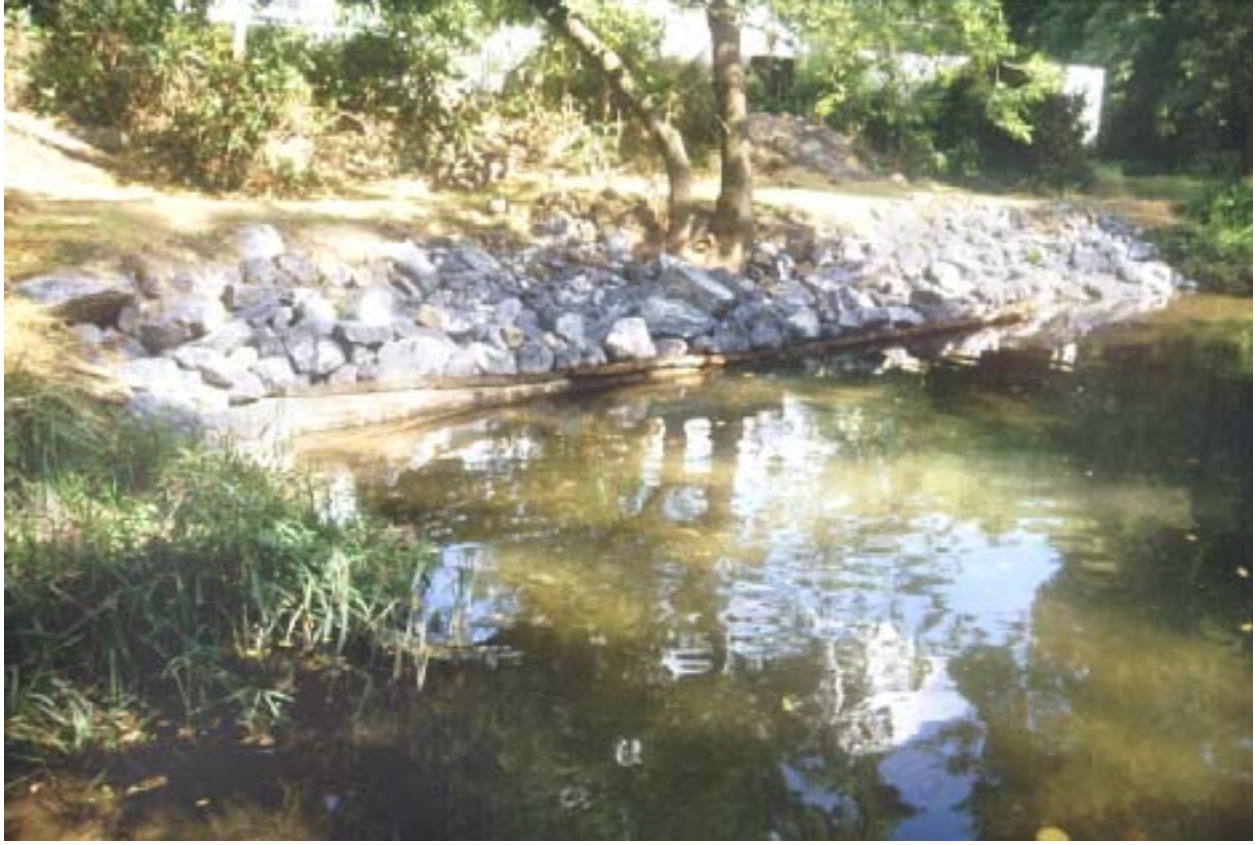
Figure 3 – Modified bank cribbing after construction. The cribbing will stabilize the eroded stream bank and provide habitat similar to that of an undercut bank.
