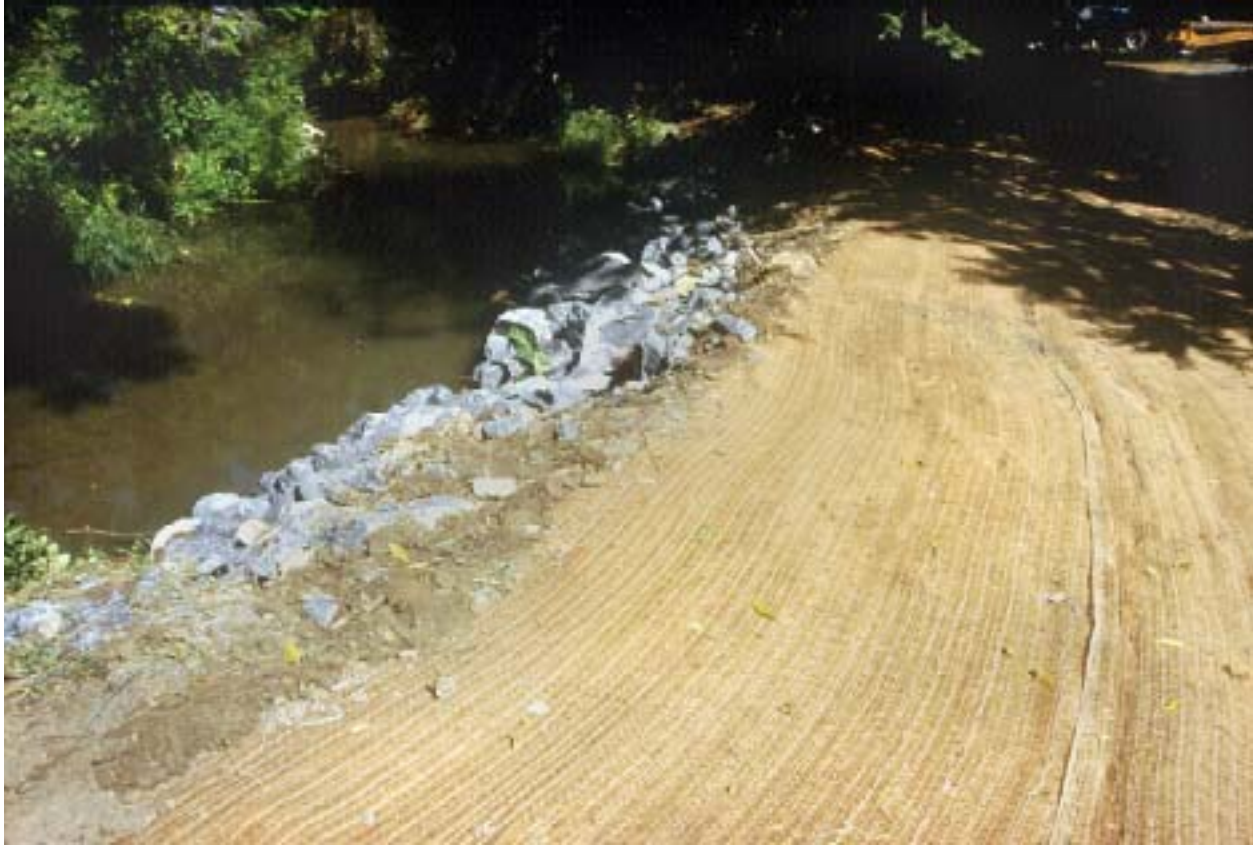
Figure 4 – Jute matting and ryegrass seed was used to re-vegetate this area behind the bank cribbing. The ryegrass will provide further bank stability during high flow episodes.
