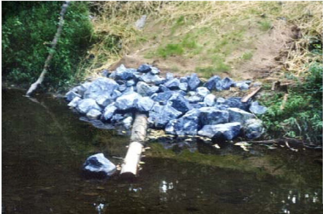
Figure 9 – Upstream single log placement. During storm events, high water will flow over the log and will be directed toward the center of the stream channel (stream flow is right to left). A sediment bar will develop against the bank downstream of the log, where vegetative establishment and channel narrowing will occur.
