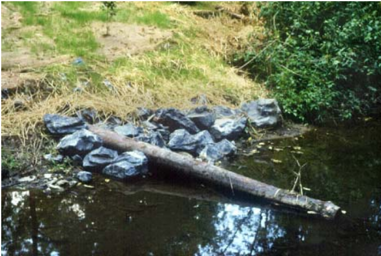
Figure 8 – A multilog deflector was installed to provide naturalistic woody habitat, direct the flow of high water away from the bank and narrow the stream channel. The bottom log was trenched low and submerged, making it difficult to see in this photo. Stone was used to secure the logs and provide toe protection, and the bank behind this device was re-graded, jute matted and seeded. Grass seed has begun to sprout through the jute matting just two weeks after construction.
