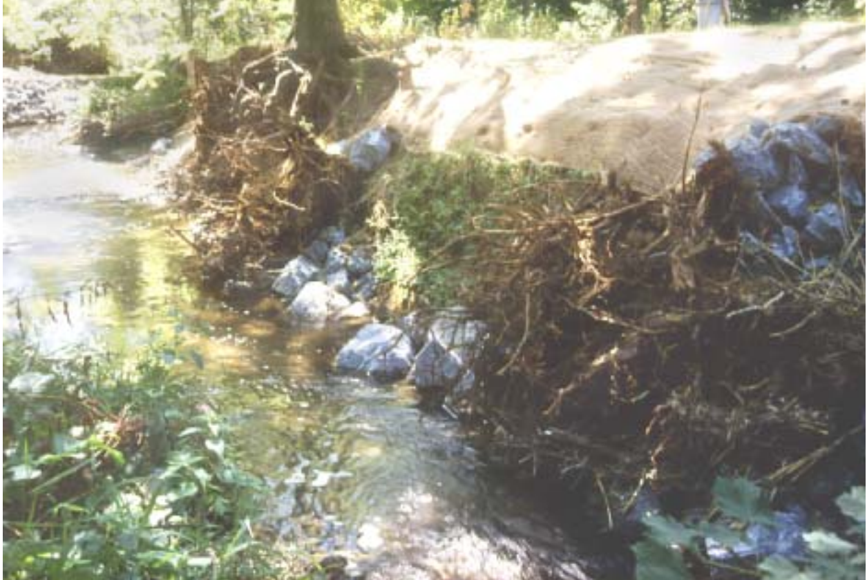
Figure 6 – Placement of root wads will direct the flow of water away from the eroded bank and toward the center of the stream channel. Stone was used to stabilize the toe of the bank and to prevent water from undercutting of the root wads.
