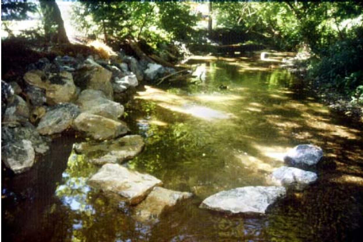
Figure 2 – Two “J-Hook” vanes were installed along the eroded section of stream bank shown in Figure 1. These devices will direct the flow of high water into a scour pool where the energy of the water will dissipate. The scour pool will also add pool diversity and provide habitat for fish. (View is looking downstream)
