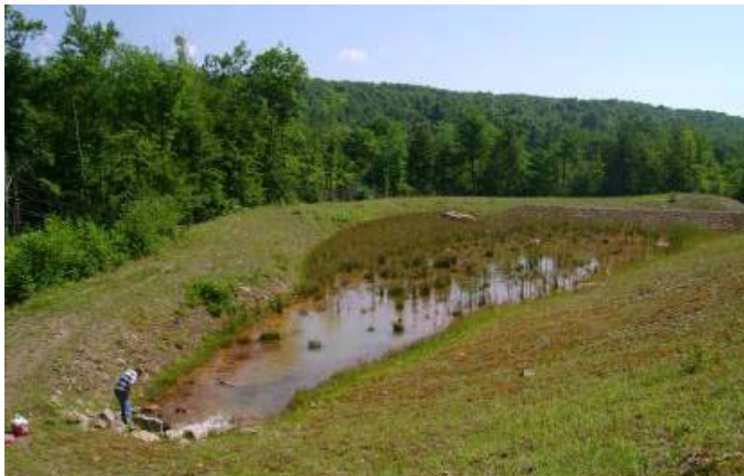
Passive Wetland Treatment System: Lausanne Tunnel water flows through pipes (forefront) into Wetland A
